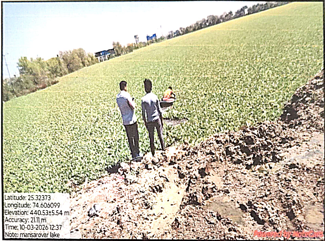
Figure 5 Manual Cleaning Work Going on at Mansarovar during Inspection
